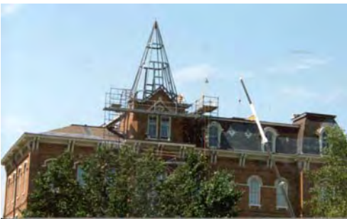
The steel frame of the tower. Photograph by Miranda Emmert
