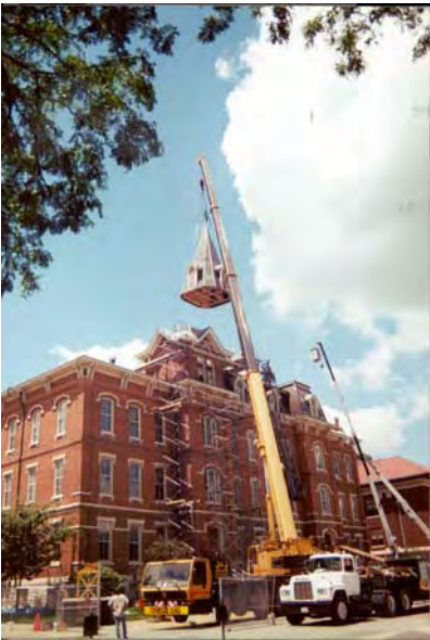
The tower being lifted. Photograph by Gordon Mork
